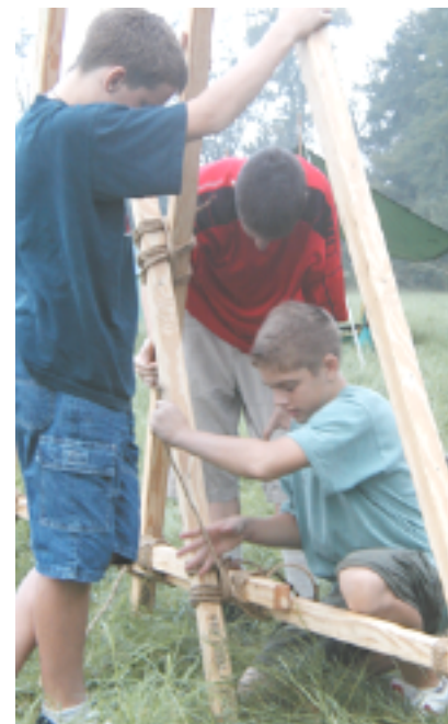
Using "Laminated Spars," Garrett Hogan lashes two A-Frames together for one side of the Double A-Frame Monkey Bridge.
