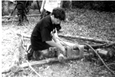
Two A-Frames are joined together to form each side of the bridge.
