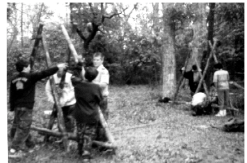
The Double A-Frames are held up in the proper positions and at the right distance.
