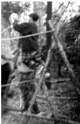
Two Hand Ropes and one Foot Rope are tied on and anchored at either end.
