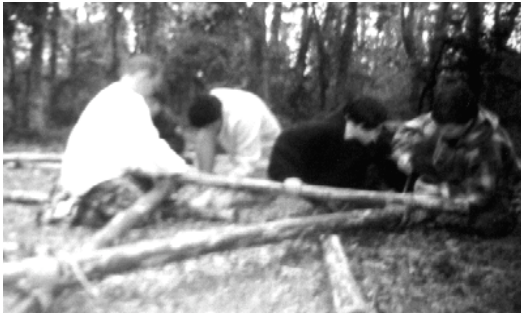
Scouts lash together two 8' spars and one 6' spar to form four A-Frames.
