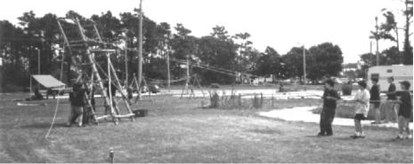
During the Carwash Fund Raiser in May of 1997, Troop 888's third 14 Foot Double Ladder Signal Tower is just about to be secured. Using rope tackles, its four 50' guylines are tied to four anchors that are already in place. Our next tower is scheduled to be built for the Troop 888 Scout Show, on Saturday, February 27 near the parking lot at St. Stephen's Church.
