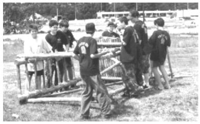
After the tower is lashed together, (which requires about 50 square lashes) it has to be carried and positioned in the exact location, before it can be hoisted.
